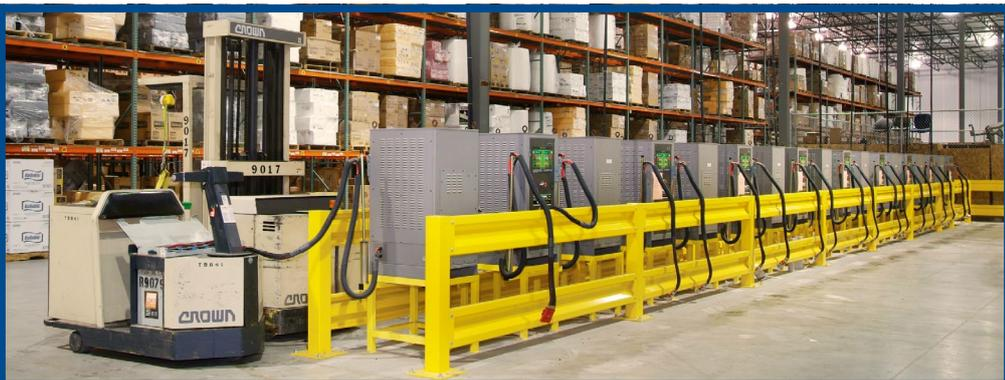
*Fast Chargers allowed International Paper to eliminate battery changes and the battery room. Lift trucks charge right where they park while operators are on break.*
